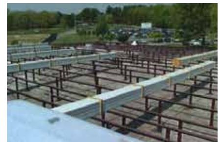
Roof under construction
