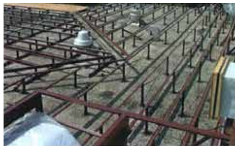
Sub-framing in place
