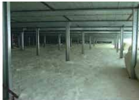
New cavity with added insulation
