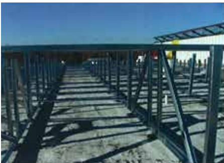
Sub-framing in place
