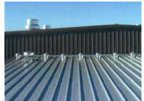
Finished metal roof
