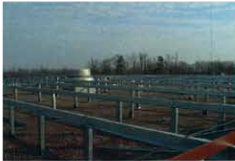
Gym with framing to add slope
