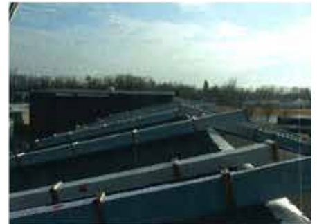
Classrooms during construction
