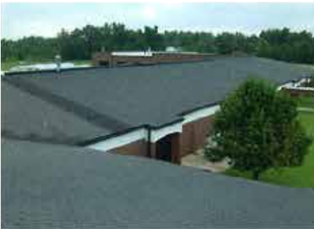
Before (Classroom-shingles, Gym-flat roof)
